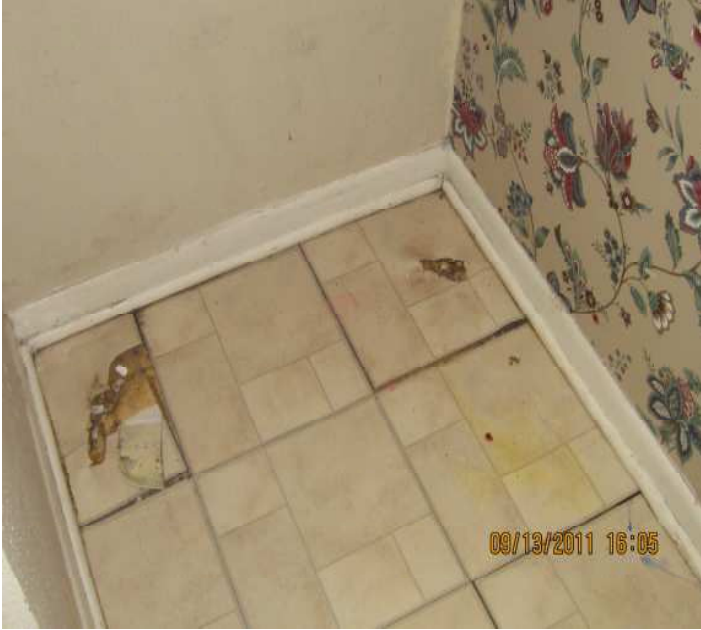
PHOTO NO. 7 DAMAGED CERAMIC TILE OVER M. BATH TUB
