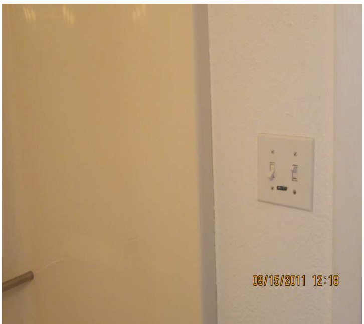
PHOTO NO. 24 WALL SWITCHES TOO CLOSE TO THIRD LEVEL BATH TUB
