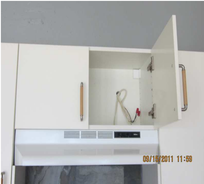
PHOTO NO. 11 LOOSE WIRING IN UPPER KITCHEN CABINET
