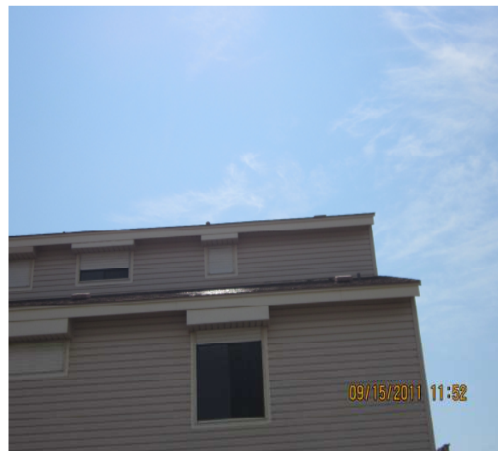
PHOTO NO. 7 FRONT SIDE ROOF SHINGLES HAVE LIFTED DURING IKE
