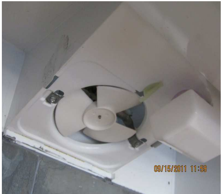
PHOTO NO. 12 KITCHEN VENT FAN MISSING A COVER
