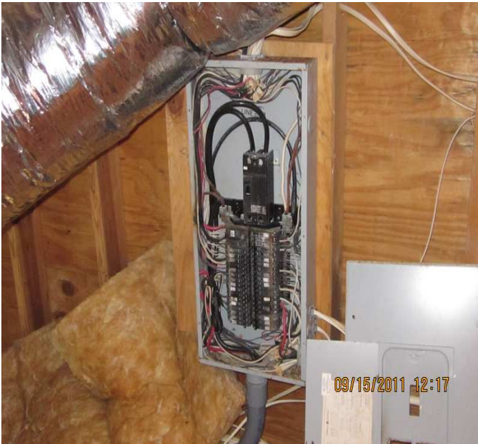
PHOTO NO. 23 BREAKER BOX IN FRONT ATTIC AREA
