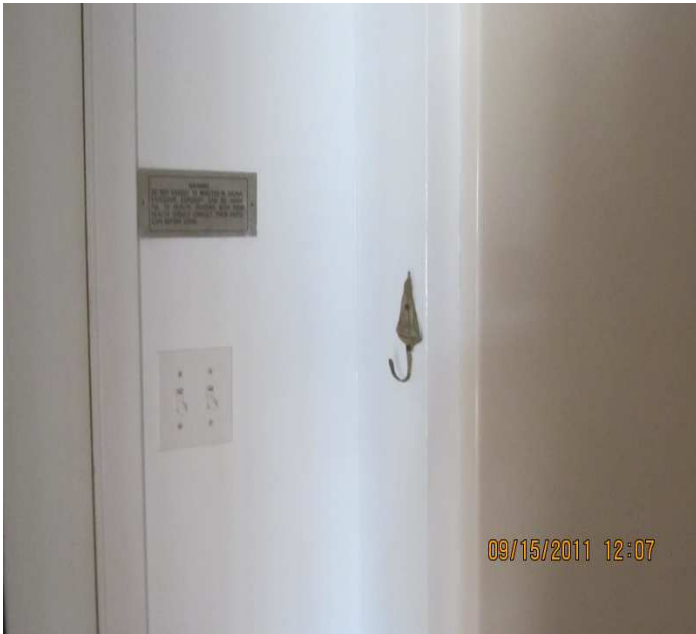
PHOTO NO. 19 WALL SWITCHES TOO CLOSE TO SHOWER IN NO. 2 BATH
