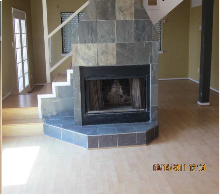
PHOTO NO. 16 LIVING ROOM STAIRWAY MISSING GUARD RAIL
