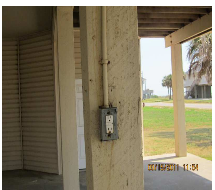
PHOTO NO. 8 EXTERIOR WALL OUTLET MISSING COVER
