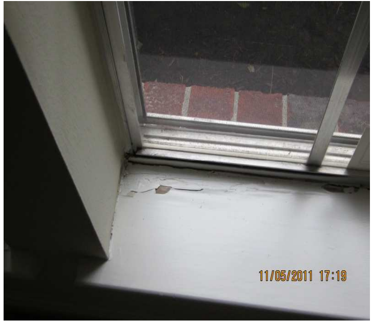
PHOTO NO. 26 WATER DAMAGED WINDOW SILL IN STUDY
