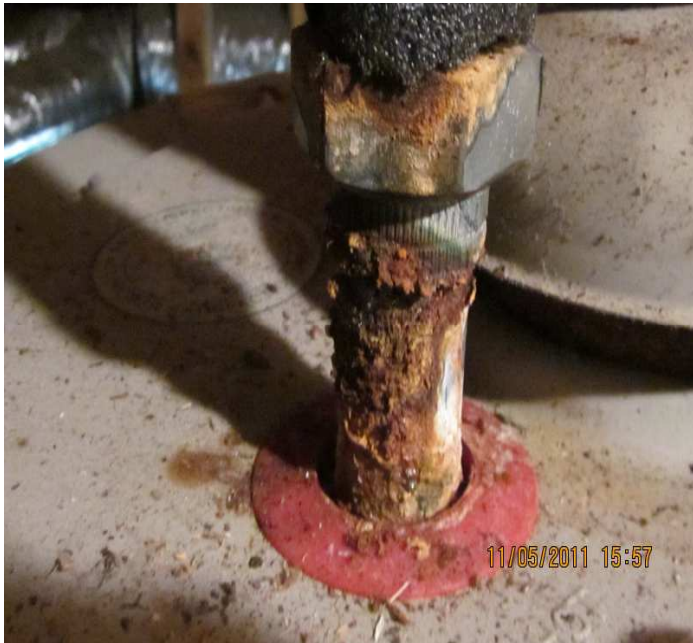
PHOTO NO. 11 BADLY CORRODED PIPING AT WATER HEATER IN ATTIC
