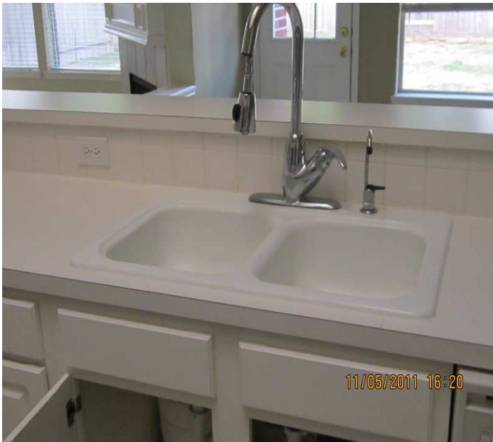
PHOTO NO. 19 KITCHEN SINK MISSING ANTI-SIPHONING DEVICE
