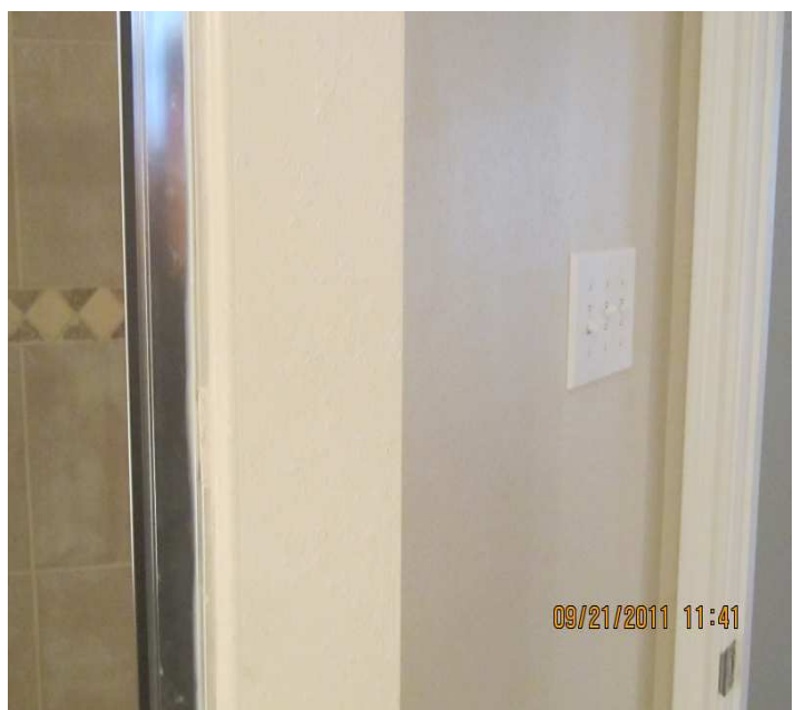
PHOTO NO. 16 WALL SWITCHES TOO CLOSE TO SHOWER IN M. BATH.
