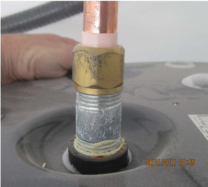
PHOTO NO. 3 WATER HEATER PIPING MISSING DIELECTRIC FITTINGS
