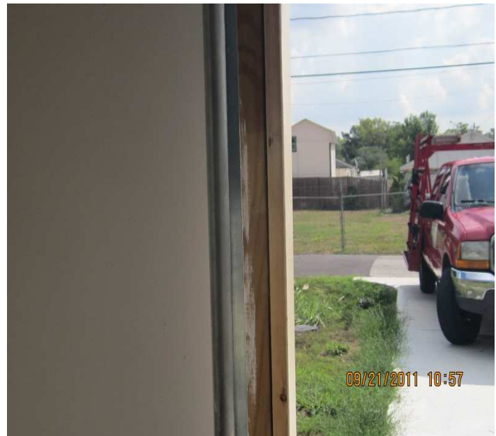
PHOTO NO. 4 VERTICAL GARAGE DOOR FRAME BOARDS NEED TO BE PAINTED
