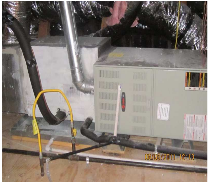
PHOTO NO. 28 INSULATION, IN ATTIC, LAYING ON VENT FAN ASSEMBLY
