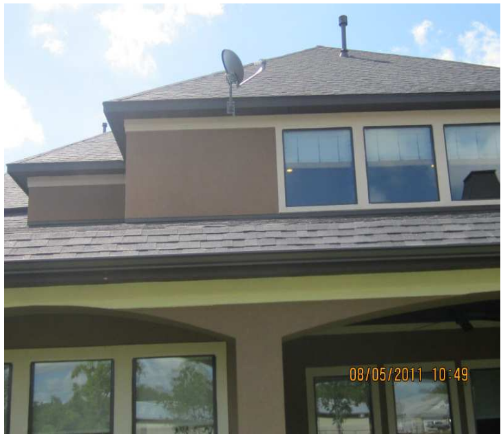
PHOTO NO. 4 TURNED UP ROOF SHINGLES ON BACK SIDE OF ROOF
