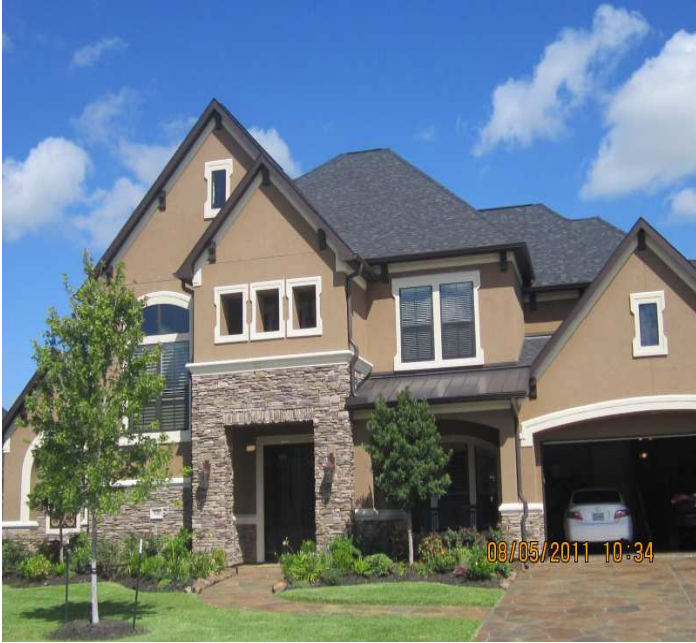
PHOTO NO. 3 MISSING GUTTERS ON WEST EAVE
