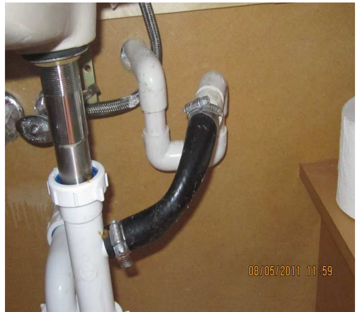
PHOTO NO. 20 BADLY CRIMPED A/C PRIMARY DRAIN LINE UNDER UPSTAIRS BATH SINK
