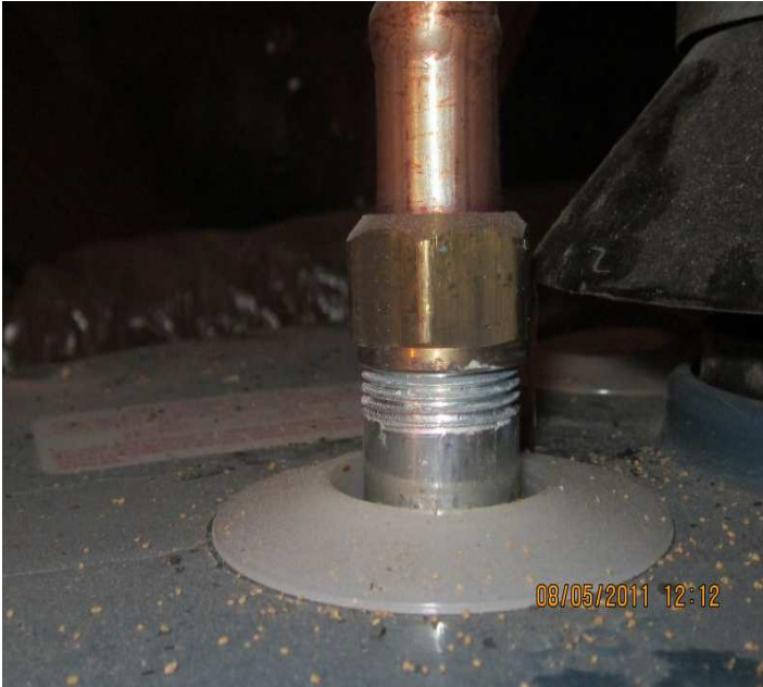
PHOTO NO. 23 WATER HEATER PIPING MISSING DIELECTRIC FITTINGS
