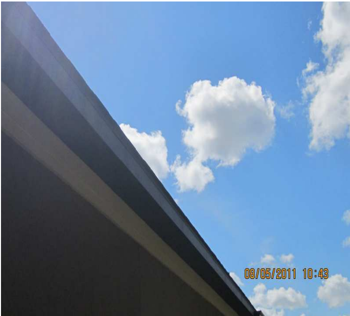
PHOTO NO. 3 MISSING GUTTERS ON WEST EAVE
