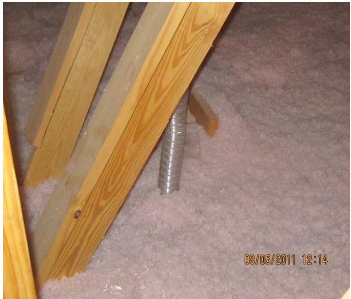
PHOTO NO. 28 INSULATION, IN ATTIC, LAYING ON VENT FAN ASSEMBLY
