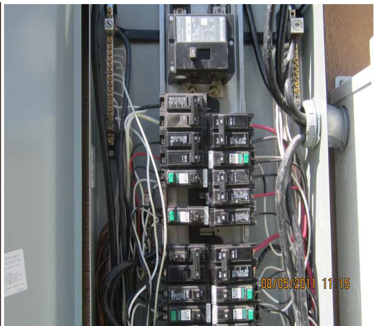
PHOTO NO. 12 200 AMP BREAKER BOX ON OUTSIDE EAST WALL
