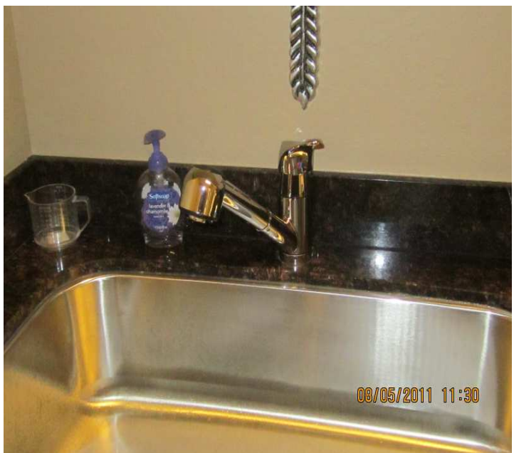
PHOTO NO. 16 UTILITY ROOM SINK MISSING ANTI-SIPHONING DEVICE
