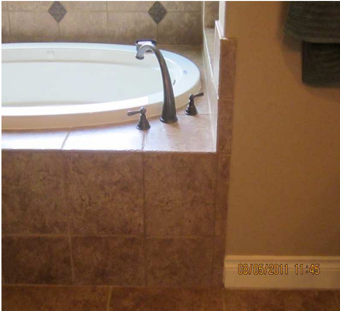
PHOTO NO. 19 TUB MISSING PLUMBING ACCESS PANEL
