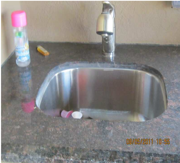
PHOTO NO. 7 BACK PATIO SINK MISSING ANTI-SIPHONING DEVICE
