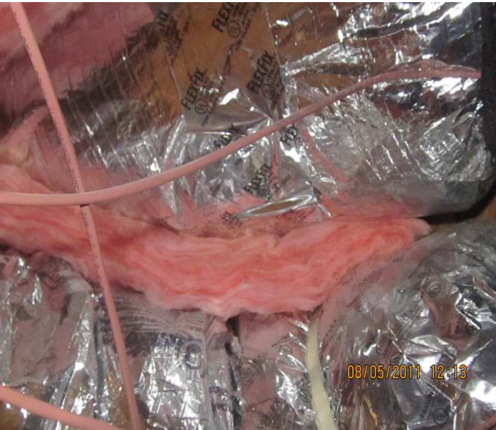
PHOTO NO. 27 PINK INSULATION BETWEEN DUCTWORK IN ATTIC
