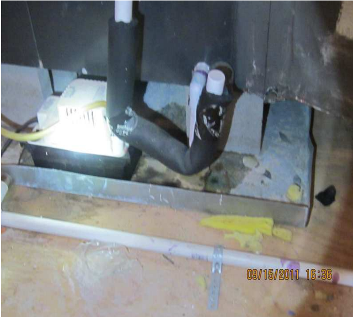
PHOTO NO. 19 A/C DRAIN PAN MISSING FLOAT SWITCH & HAS WATER IN IT.
