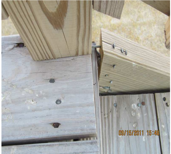
PHOTO NO. 8 DAMAGED WOOD PIER IN BACK
