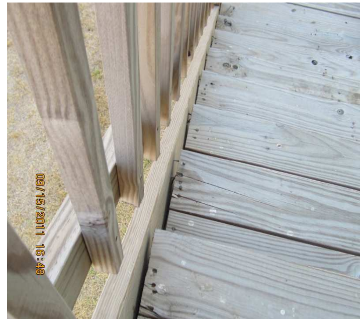
PHOTO NO. 20 STEPS, ON EXTERIOR STAIRWAY, PULLING APART
