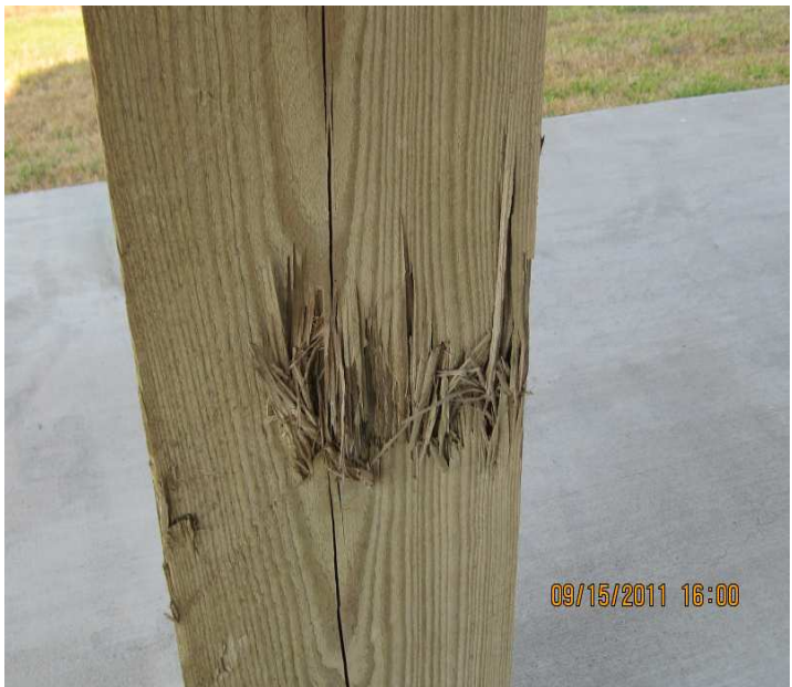
PHOTO NO. 8 DAMAGED WOOD PIER IN BACK
