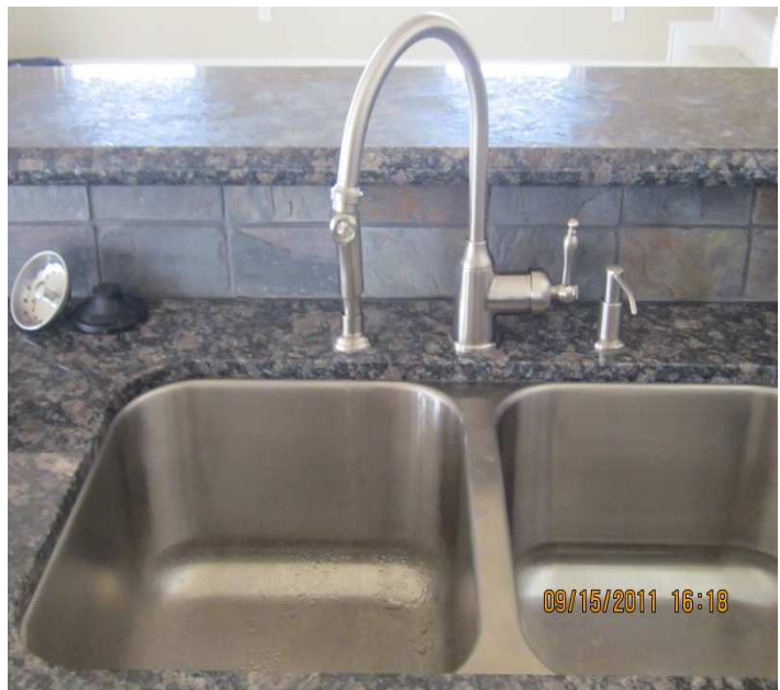
PHOTO NO. 12 KITCHEN SINK MISSING ANTI-SIPHONING DEVICE
