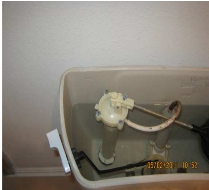
PHOTO NO. 7 COMMODE TANKS MISSING ANTI-SIPHONING DEVICE
