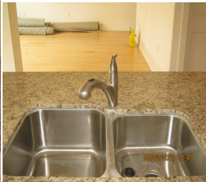
PHOTO NO. 4 KITCHEN SINK MISSING ANTI-SIPHONING DEVICE
