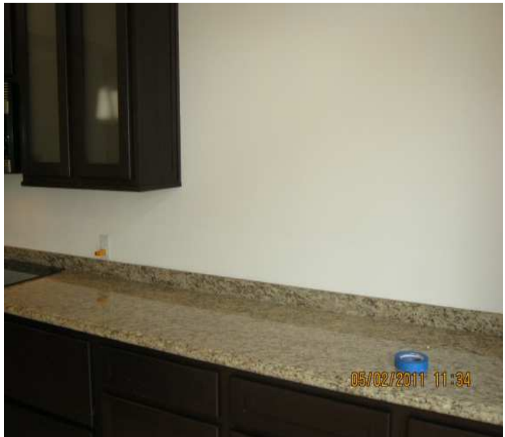
PHOTO NO. 12 EAST SIDE KITCHEN COUNTER TOP, NEEDS ADDITIONAL OUTLET S
