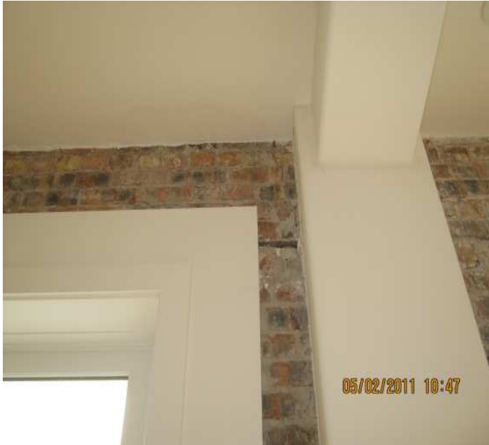
PHOTO NO. 3 DAMAGED BRICK MORTAR ON EAST LIVING ROOM WALL
