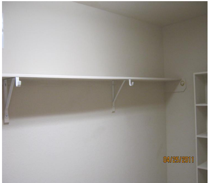
PHOTO NO. 20 CLOSET POLES NOT INSTALLED
