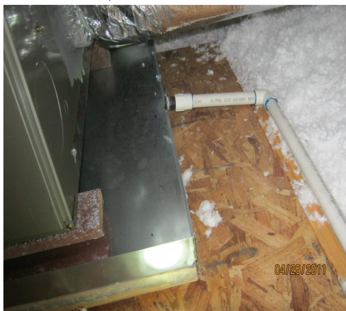
PHOTO NO. 16 METAL A/C DRAIN PAN, IN ATTIC, MISSING FLOAT SWITCH
