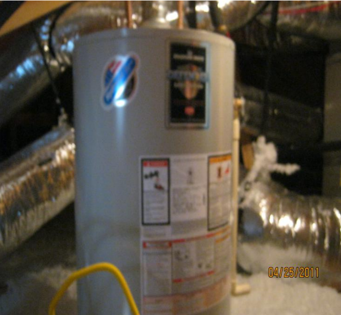
PHOTO NO. 15 GAS WATER HEATER IN ATTIC
