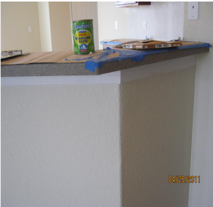
PHOTO NO. 23 WALL, UNDER KITCHEN COUNTER TOP, NOT ALIGNED PROPERLY
