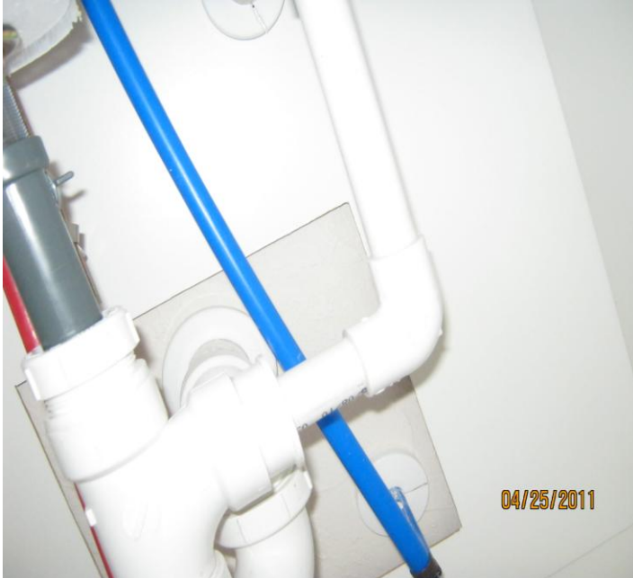
PHOTO NO. 23 WALL, UNDER KITCHEN COUNTER TOP, NOT ALIGNED PROPERLY
