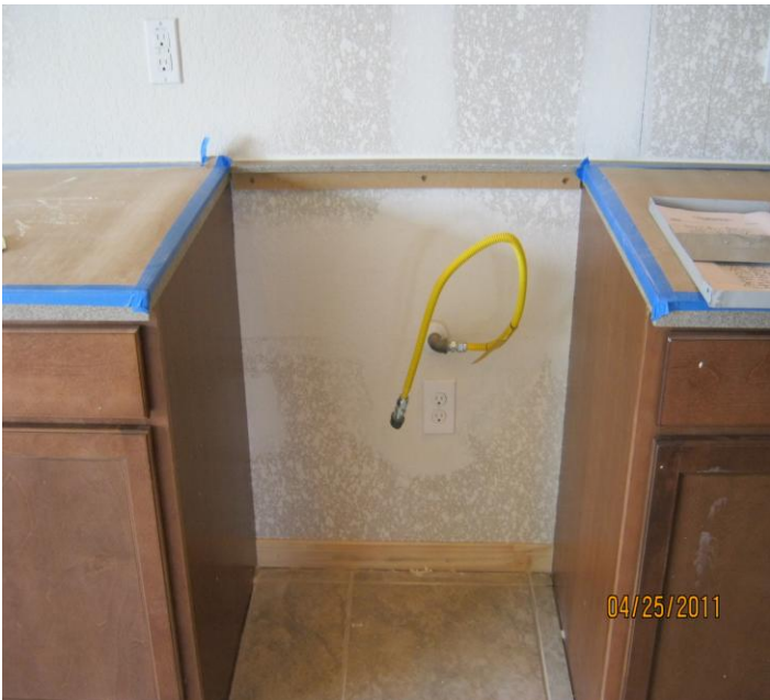
PHOTO NO. 19 GAS LINE, TO RANGE, IS NOT EASILY ACCESSIBLE
