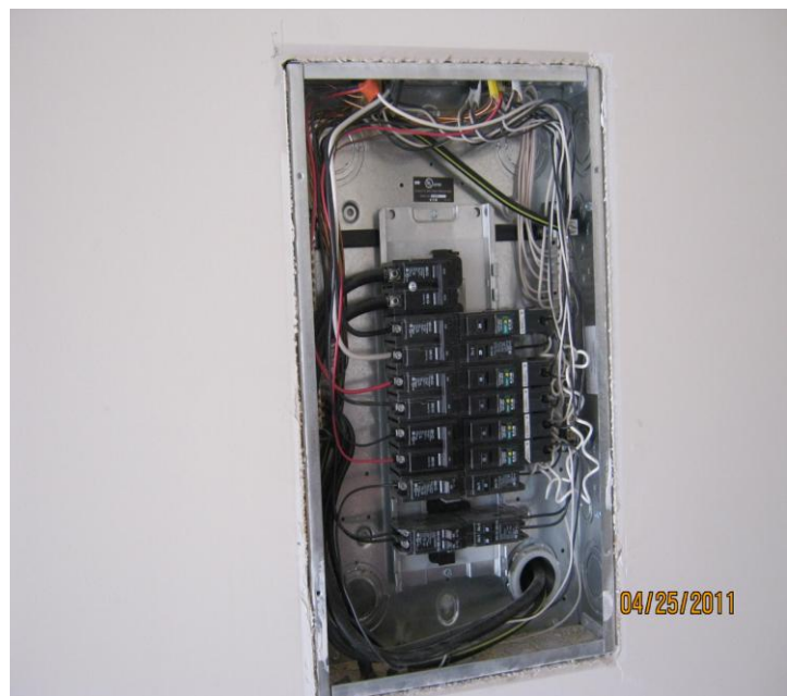
PHOTO NO. 12 BREAKER BOX INSIDE GARAGE
