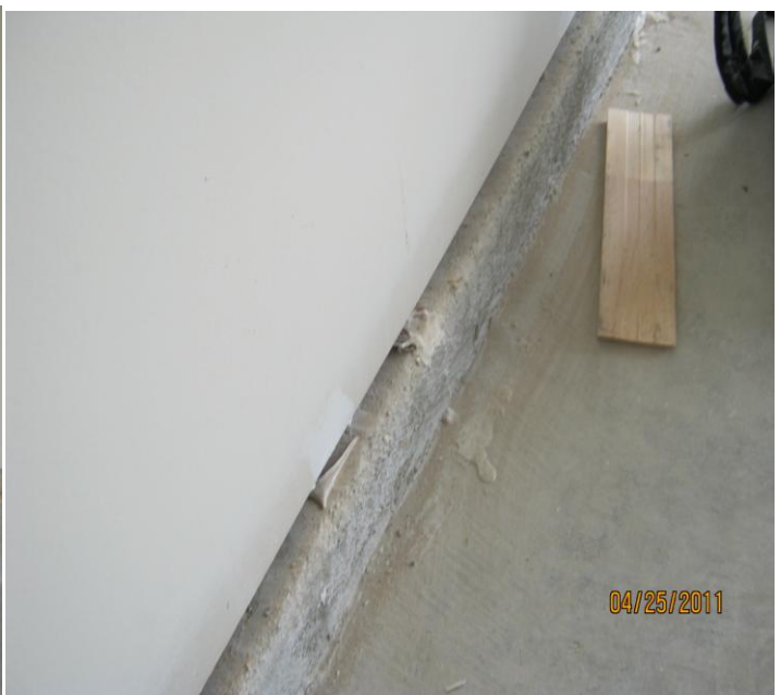
PHOTO NO. 4 DAMAGED INTERIOR GARAGE WALLS & GAPS
