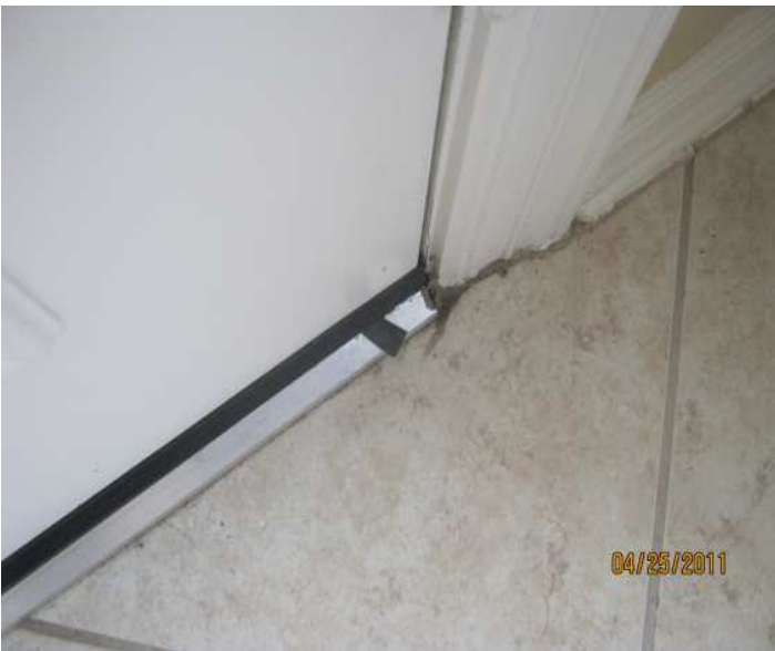
PHOTO NO. 23 DAMAGED WEATHER STRIPPING AT BOTTOM OF BACK EXIT DOOR
