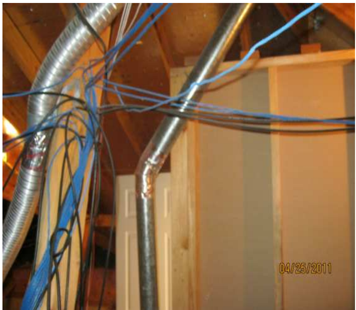
PHOTO NO. 20 VERTICAL METAL DRYER VENT IN ATTIC
