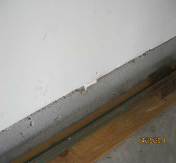
PHOTO NO. 23 DAMAGED WEATHER STRIPPING AT BOTTOM OF BACK EXIT DOOR
