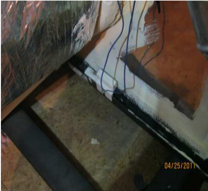
PHOTO NO. 19 A/C DRAIN PAN, IN ATTIC, IS TOO SHALLOW
