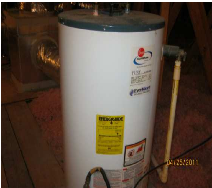
PHOTO NO. 16 GAS WATER HEATER IN ATTIC
