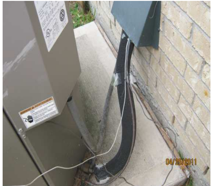
PHOTO NO. 12 GAPS, AT A/C HOSES BY CONDENSER UNIT
